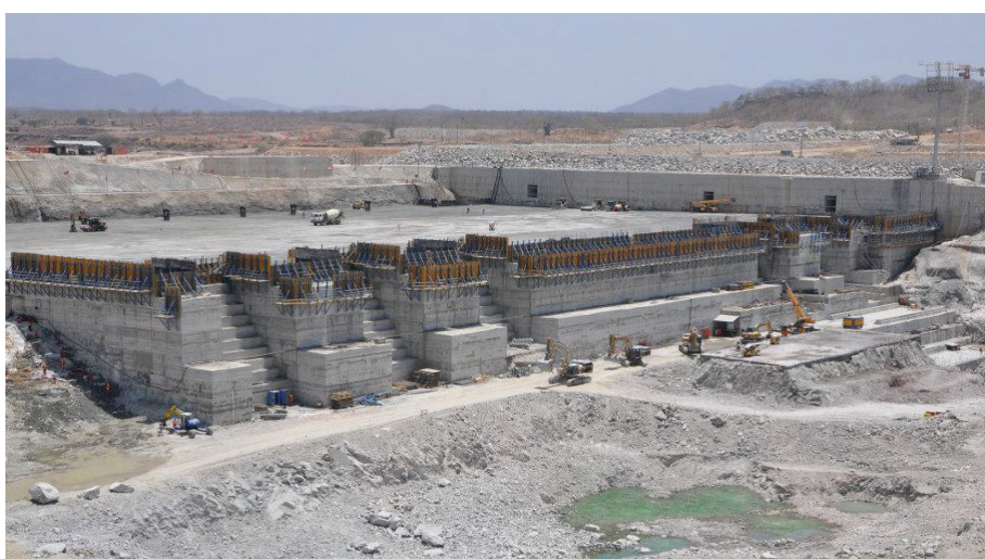
The Great Renaissance Dam under Construction
