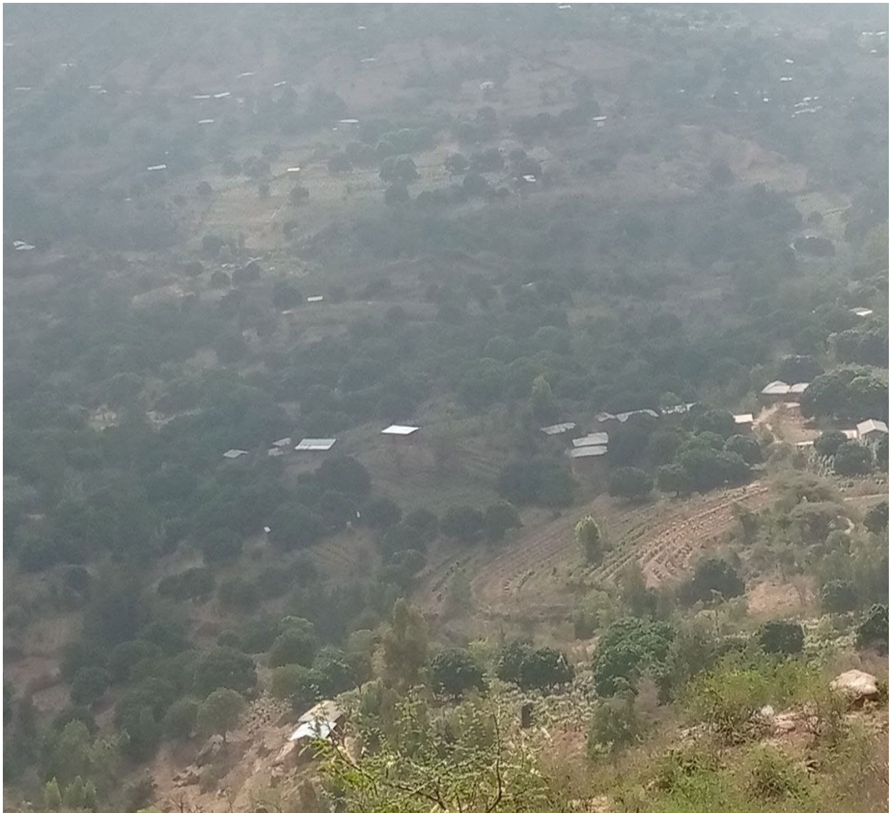
Figure 8: Watershed activities in the lower catchment of residential area
