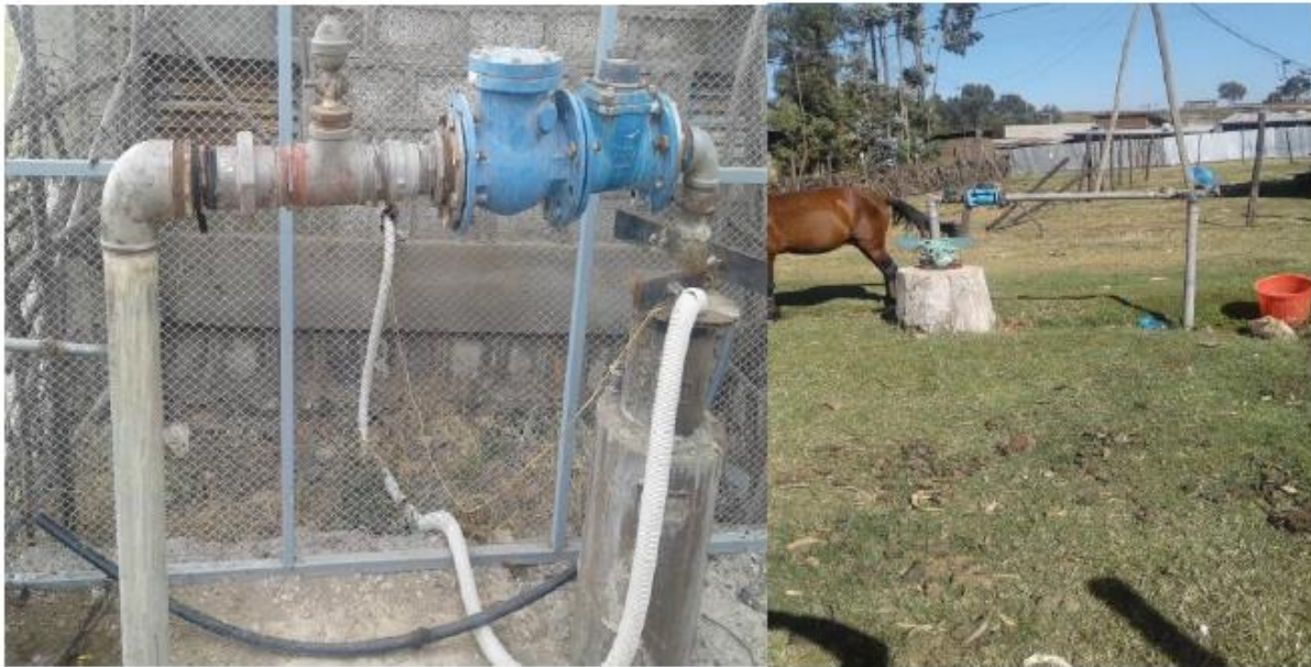
a) Borehole of Wale b) Borehole of Kera around
